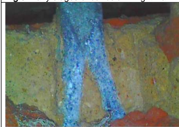
Fig 9: Early stages of corrosion – right wall.
